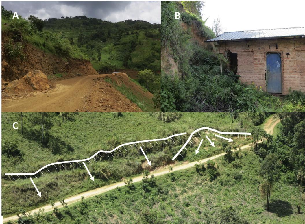
Fig. 10. Failures along a newly constructed road (Kabonero, October 2014) (A, C), Failure of a cut in the hillslope for the construction of a house (Mahango, September 2014) (B).
